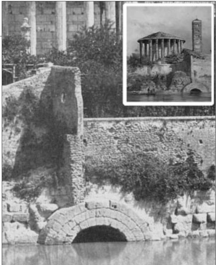
Two views of an entrance to the Cloaca Maxima. This sewer system was built around 750 BC and is still in use today.
